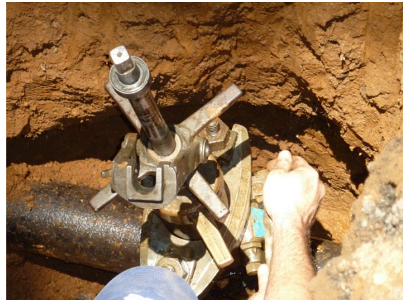
Getting ready to thread in one of the shutoffs.
