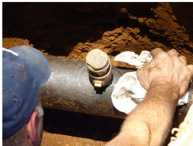
Admiring a job well done!
